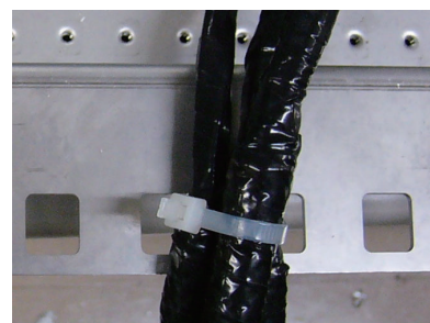
Fix cables to post with cable tie
